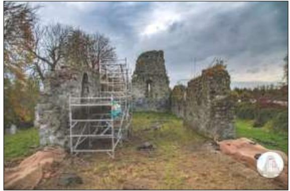
What's left of the walls of this medieval church, are being pointed and repaired in the hope that they will withstand the elements for a long time to come.
